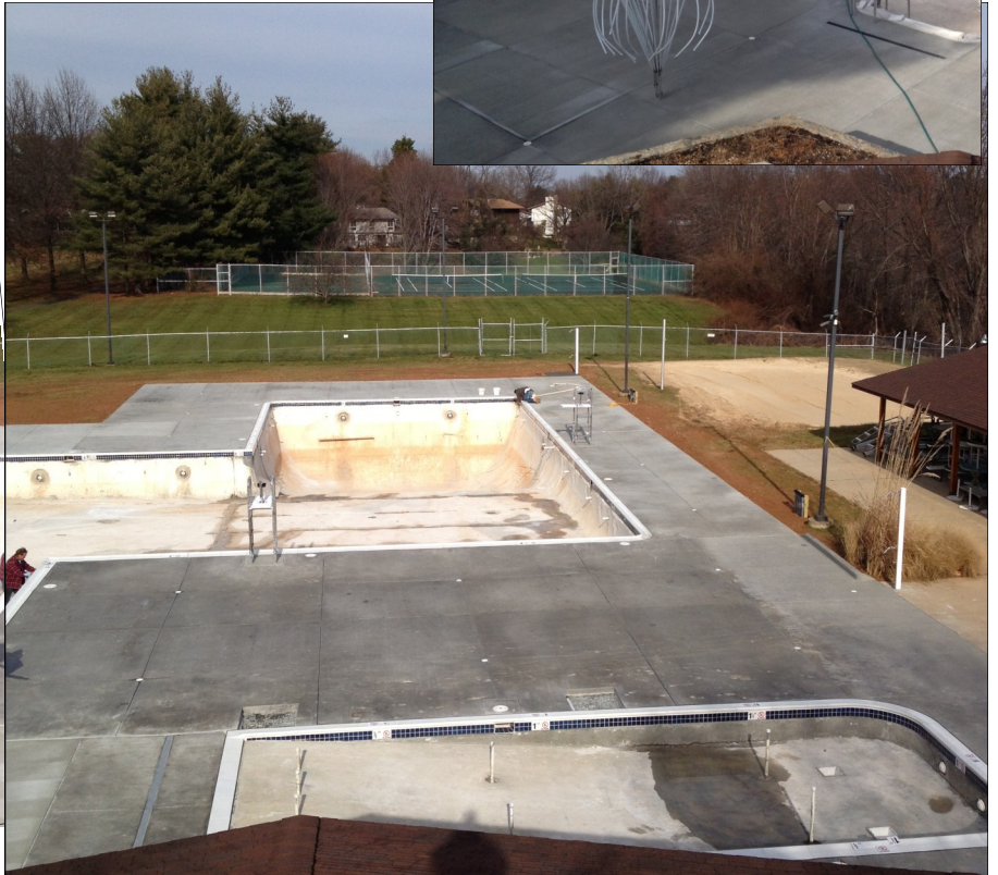
OVERVIEW OF POOL WITH NEWLY POURED CONCRETE POOL DECK, NEW BABY POOL (notice new, graduated slope), and NEW COPING TILES IN PLACE (i.e., tile around all pool edges). MAN INSIDE POOL WORKING ON TILES.
