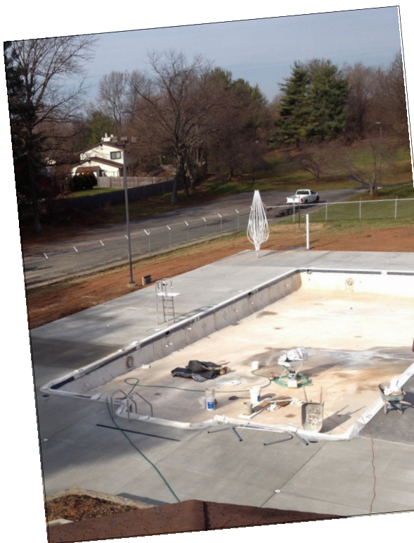
OVERVIEW OF POOL WITH NEWLY POURED CONCRETE POOL DECK, NEW BABY POOL (notice new, graduated slope), and NEW COPING TILES IN PLACE (i.e., tile around all pool edges). MAN INSIDE POOL WORKING ON TILES.
