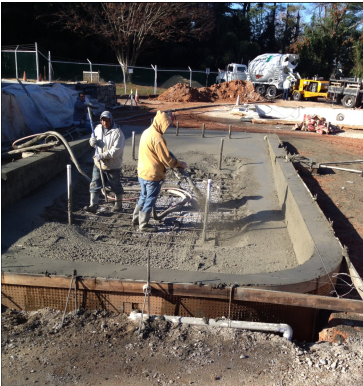
NEW CONCRETE BEING POURED FOR BABY POOL
